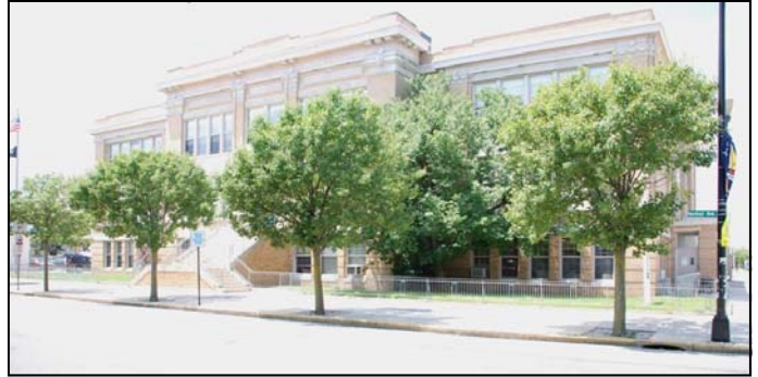
Old Richmond Avenue School before demolition (photo courtesy of the Atlantic City Free Public Library)
